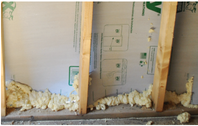
Fiber board requires a lot of material to seal edges and joints due to the thin and flexible nature of the board.
